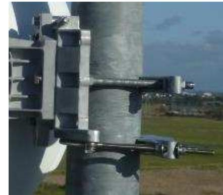
+/- complex azimuth and elevation tuning
